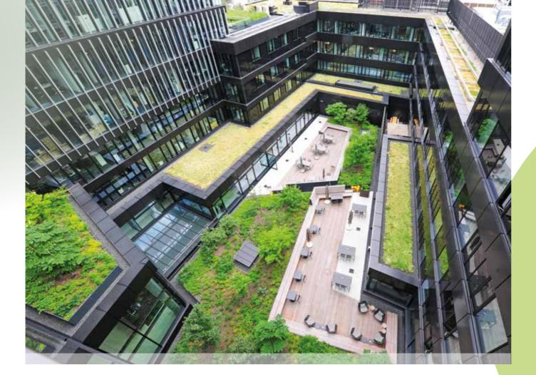
Green roofs are installed on top of existing roof spaces. These spaces are then protected from UV radiation in the summer and from frost in the winter. The protective layer also acts as additional thermal insulation – heating and cooling the inside of the building depending on the time of year. However, roof planting not only enhances the structural fabric
