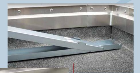
Bend the upper frame section at the perforation and hook it into the slot on the lower section.
