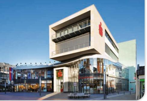
Different facade sections, whether round or straight, are all edged with custom-made channels and gratings.
