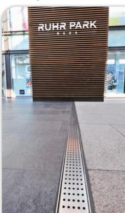
20,000 m2 of the open-air space in Ruhr Park Bochum was relaid with different-coloured granite. The channels were often laid as a visual dividing line directly between the different-coloured slabs.
