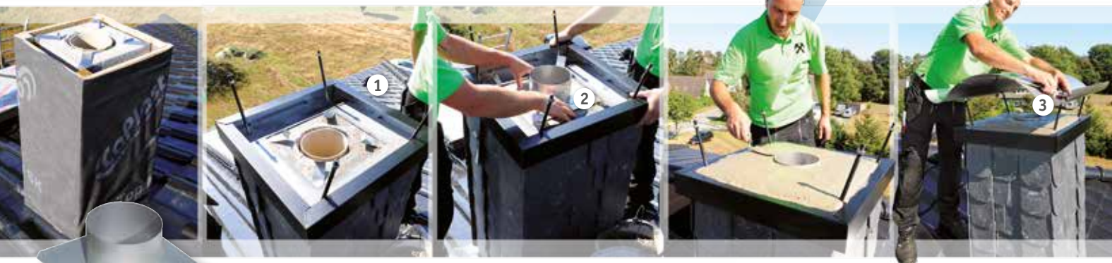
Step 1: Fitting the shuttering frame
