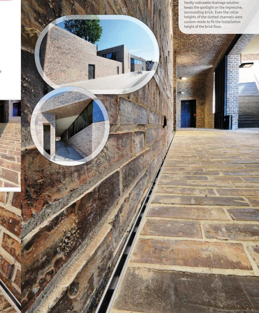
The slotted channels discreetly sneak along the rough stone brick walls. This
