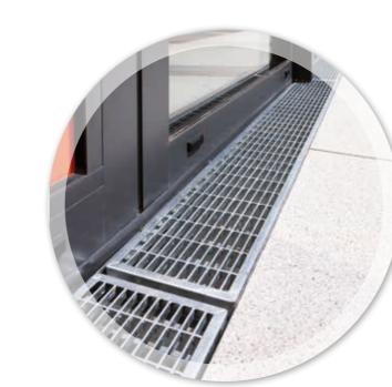
Drainage systems and mesh gratings made of hot-dip galvanised steel ensure proper dewatering in front of the glass facade of the school's canteen and the access to the kitchen.
