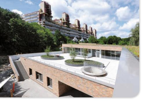
The drainage and dewatering systems surround the entire courtyard. The building's overall look of robust, hot-dip galvanised steel elements is created by the rails, safety lattice for the overhead lights and even the dewatering systems including their mesh gratings.
