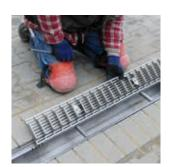
Precisely place the gratings with the locking mechanisms on the channels. Depending on the grating type, the locking mechanisms may be enclosed loose with the product and need to be installed in situ.
