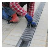
Carefully lock the gratings in place. Ensure that the bolts reach under the cross bars.
