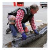
The channels can be interlinked using the pegs. To do so, place the channels on the pegs at an angle of approx. 45 degrees and then slowly tilt them downwards.
