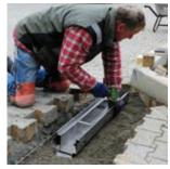
Prepare the foundation for the channel and place the channel at the appropriate height.
