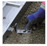
Now mount the concrete anchor. The shape of the anchor may vary depending on the height of the channel (straight/angled)
