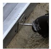
Then connect the channel elements using the screw connections still to be affixed.
