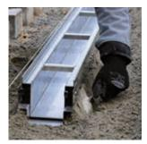
Ensure that the black plastic elements are fully lined as these bear the loads through to the foundation.
